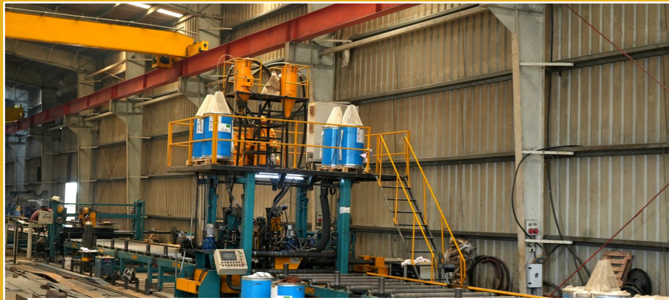
Line-1 PHI & Assembly with automatic welding machine (SAW).
